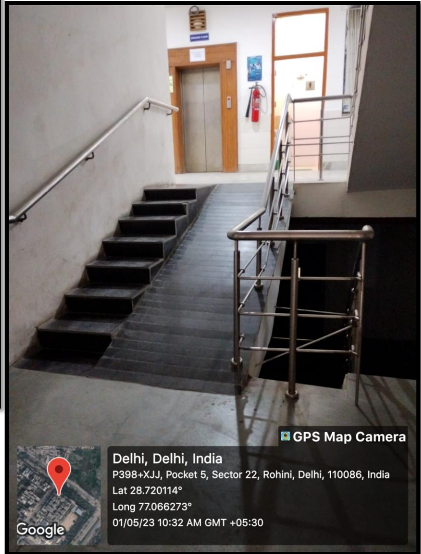
Ramp and Lift at the entrance of the 7th Block
