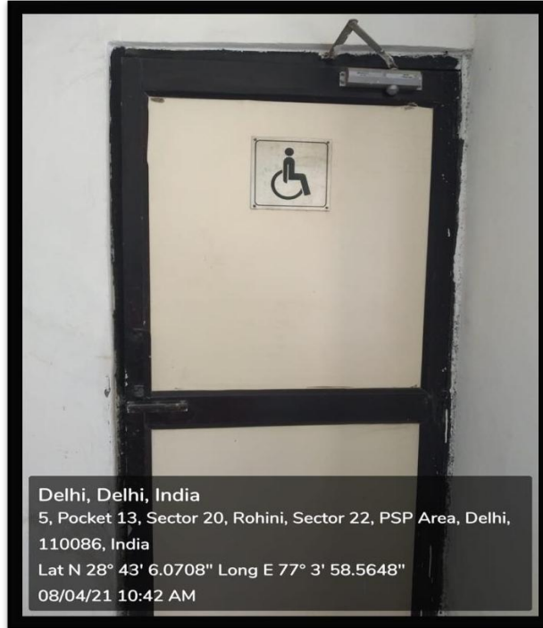
Disabled Friendly Washrooms
